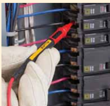
Reduce tip exposure for CAT III testing
